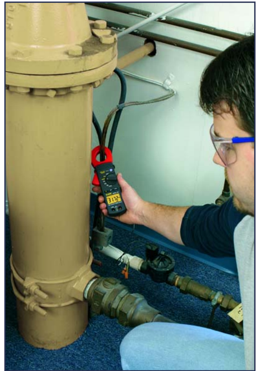
Measuring leakage current on a ground wire with the TRMS Leakage Current Meter Model 565
