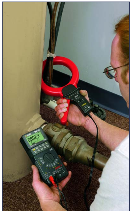
Model 2620 checking for ground fault currents
